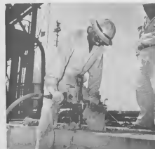
DOWELS FORMED in greenheart are inserted in the Carpenter Shop and then driven into openings in new timbers where bolts had been driven through. Glued and sawed flush, the result is a closed, smooth finish on the timber's outside side. This was done 4000 times along the length of the pier.
